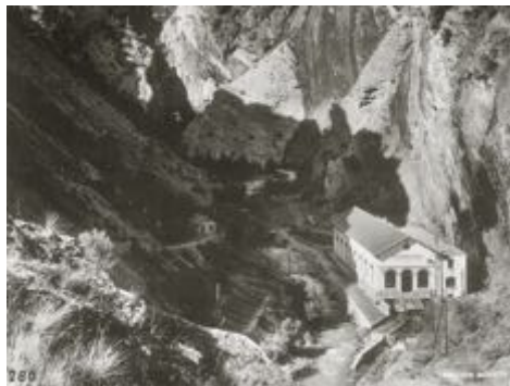
Hydroelectric plant Gampel 1898
